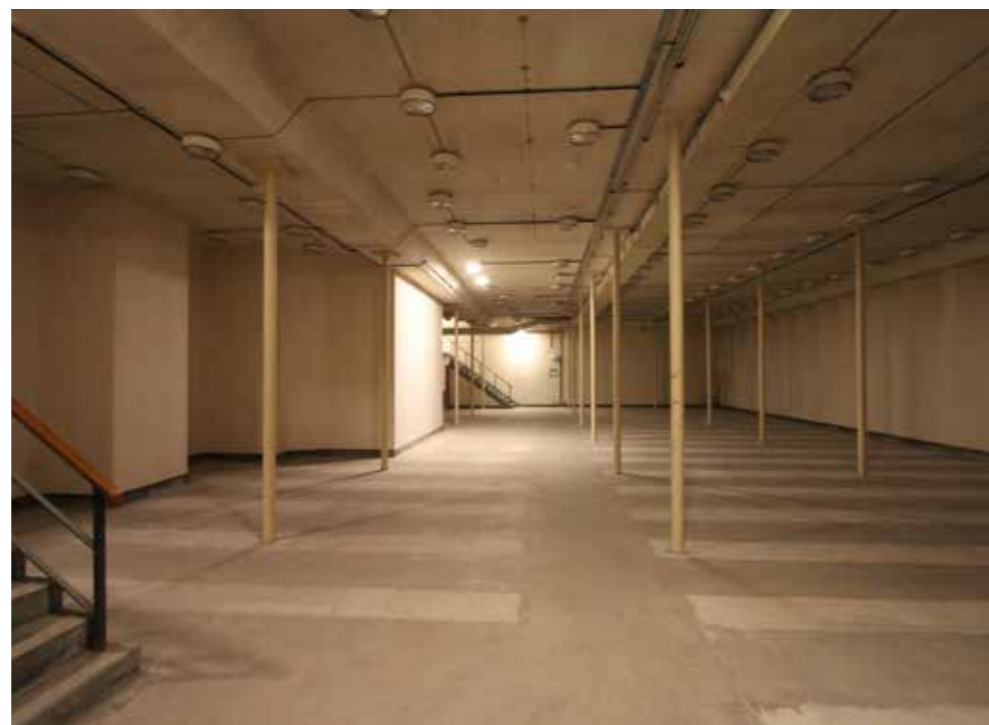
Existing lower basement of Rhodes House
