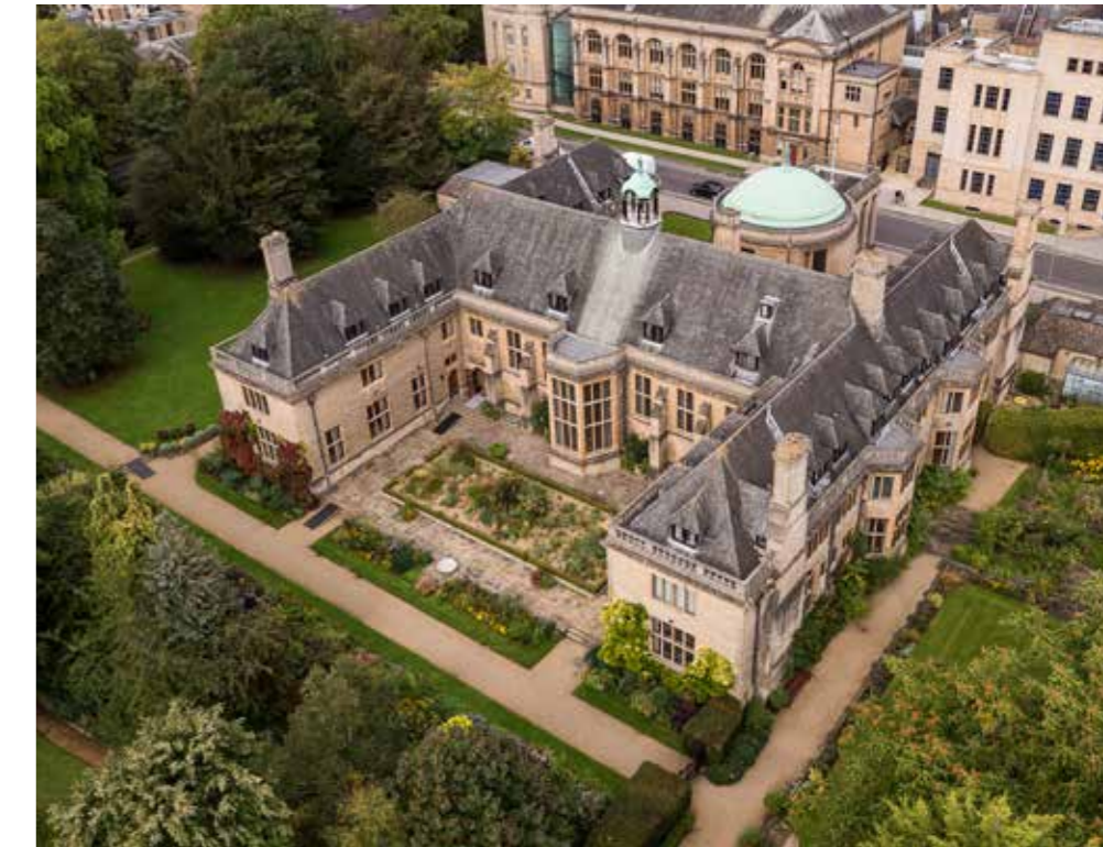
Aerial view of Rhodes House from the Southeast
