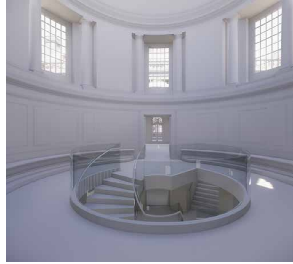
Study for the spiral stair in the Rotunda - Note; balustrades shown indicatively as glass to show the height required
