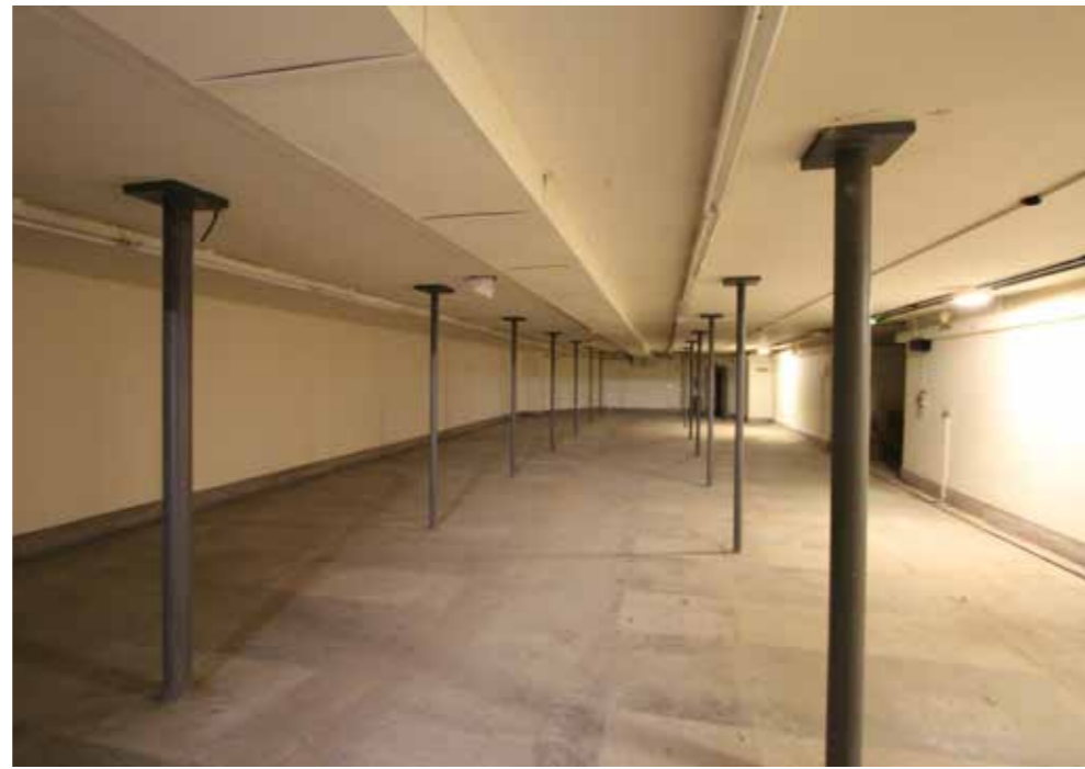
Existing upper basement of Rhodes House
