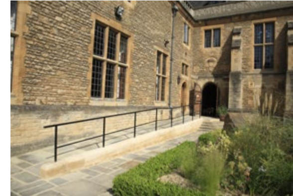
Rhodes House access ramps
